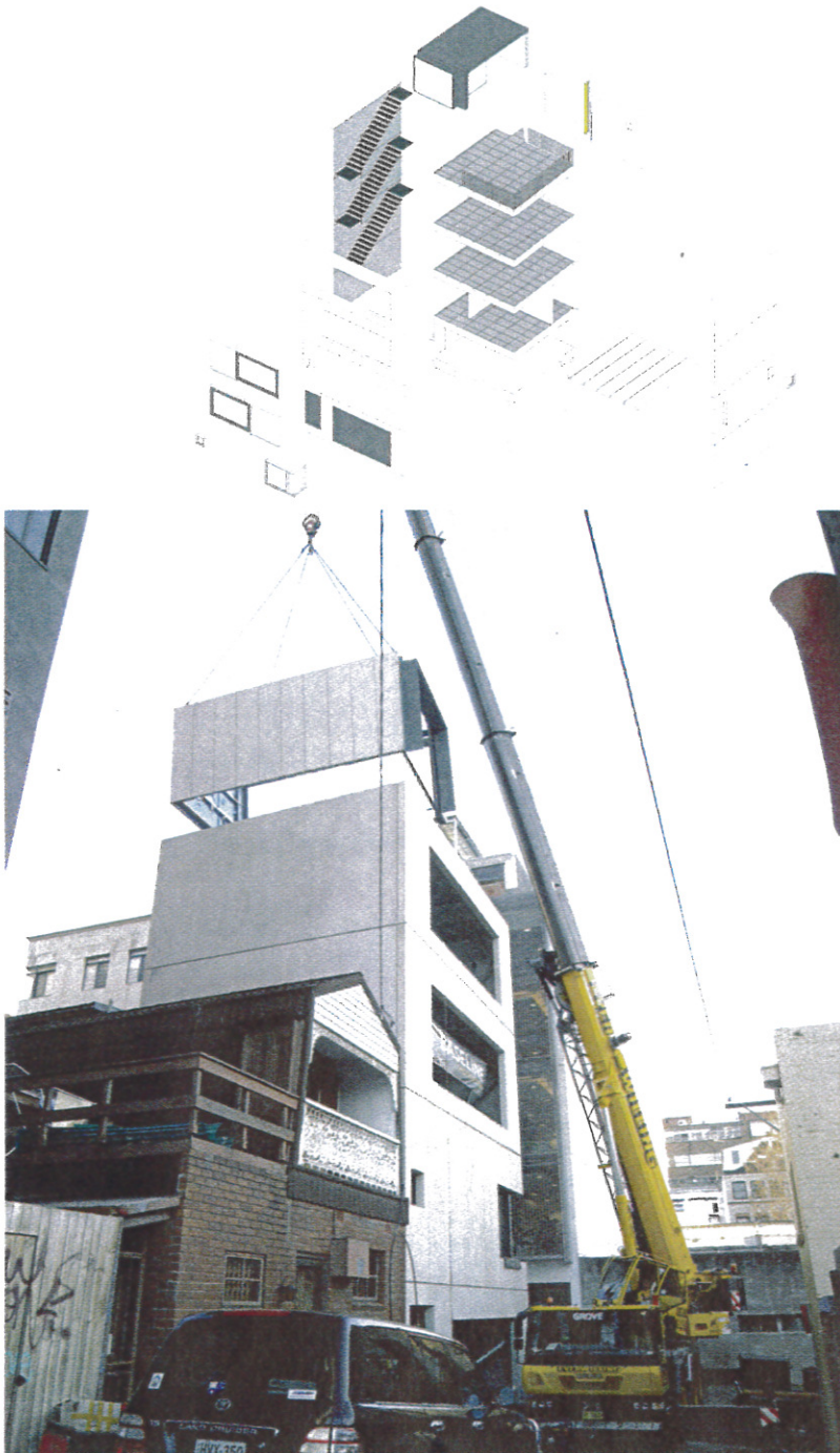
Top left: 'Exploding' diagram showing precast elements to the building.
