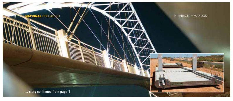
bridge sections together. The bridge segments were held by temporary cables during this operation. As soon as the arch was joined, the 300mm thick precast decking units were sequentially placed – each being bolted to the steelwork and the previous unit using a steel bracket with a box-out to conceal the fixing. Next, prestressing strand was threaded through each edge of the deck and grouted to enhance resistance to the cyclonic wind uplift forces.
