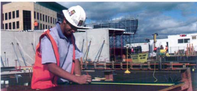
Aaron Marr civil construction carpenter working at the Australian Technology Park.
