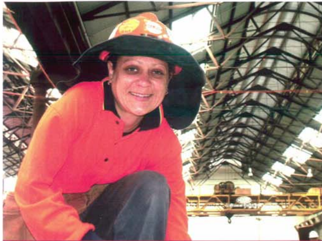
Alana Varga, St Hilliers first female carpentry apprentice, at work on the North Eveleigh site.
