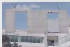
Large wall panel being erected
